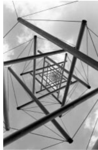
Figure 4.26: Sometimes trusses are used only because they look nice. The tensegrity structure 'Needle Tower' was designed by artist Kenneth Snelson and is on display in the Hirshhorn Museum in Washington, DC. Here you are looking straight up the middle. Photograph by Christopher Rywalt.
