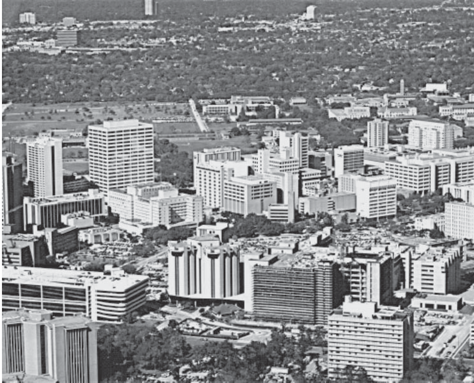
EXPOSURE B STRUCTURES IN THE FOREGROUND ARE LOCATED IN EXPOSURE B. STRUCTURES IN THE CENTER TOP OF THE PHOTOGRAPH ADJACENT TO THE CLEARING TO THE LEFT, WHICH IS GREATER THAN APPROXIMATELY 656 FT (200 M) IN LENGTH, ARE LOCATED IN EXPOSURE C WHEN WIND COMES FROM THE LEFT OVER THE CLEARING. (SEE FIGURE C26.5-2.)
