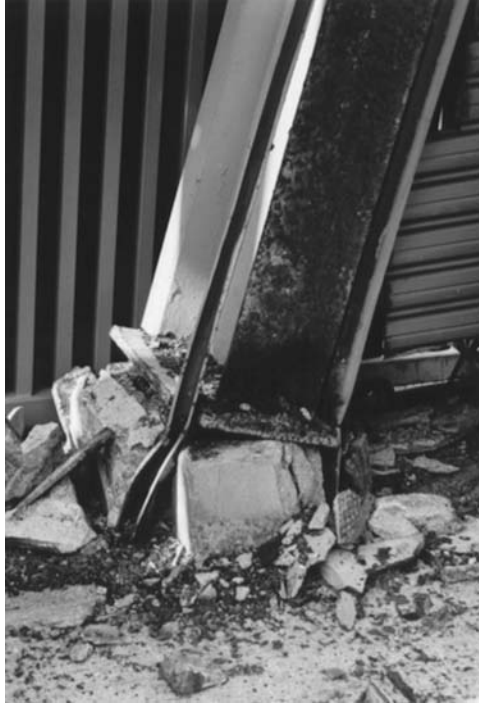
FIGURE 9.44 Example of failed column base connection.
