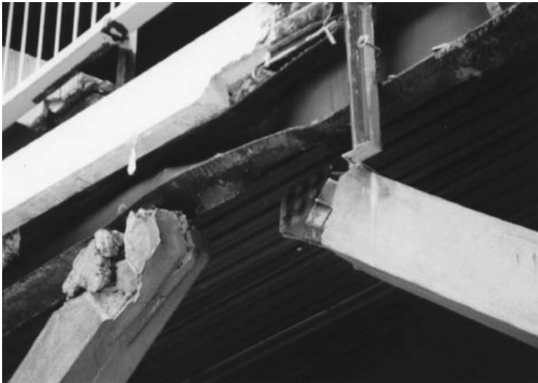
FIGURE 9.36 Inelastic rotation at brace connection point in absence of lateral bracing.
