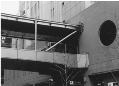
FIGURE 9.45 Failed brace anchorage.
